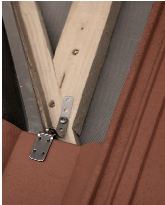
512 secures cut tile in the valley.
