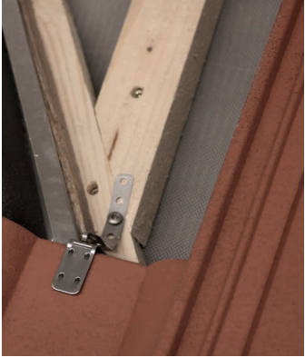
512 secures cut tile in the valley.
