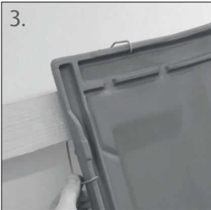
3. Place lower end of the clip onto the sidelock of the tile.
