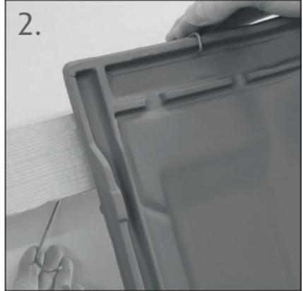
2. Guide the clip from the top behind the batten. Place upper end of the clip onto the headlock of the tile.
