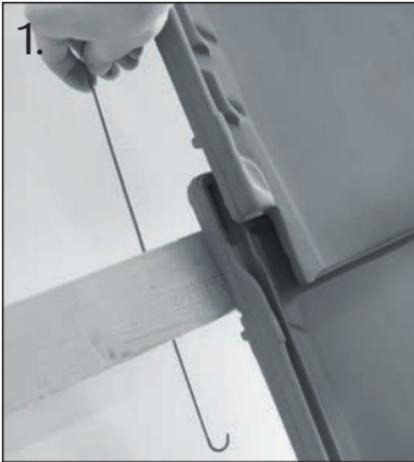
Hold the clip at the top and slide behind the batten.
