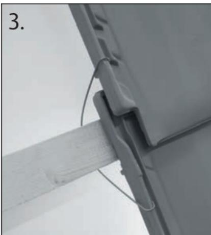
Secure the bottom end of the clip onto the sidelock to another tile.
