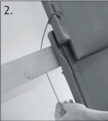
Secure the top of the clip onto the sidelock as close to the batten as possible.
